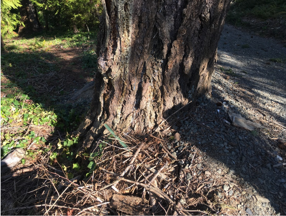
Figure 6. Common root plate condition of trees along gravel drive (Photo taken March 22, 2019).
